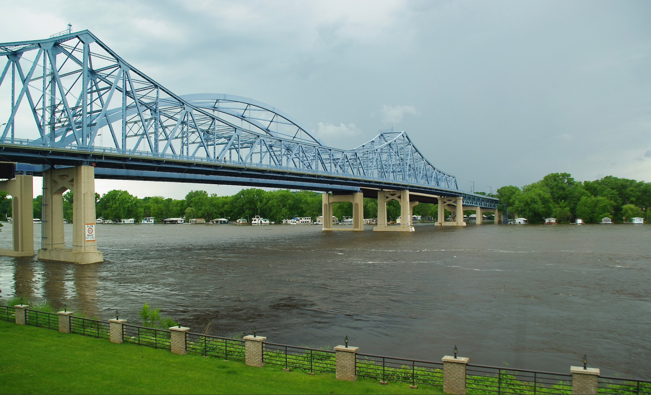
This bridge is historic and rare, a cantilever through truss bridge, stretching westbound across the Black River to the Mighty Mississippi, from La Crosse to Barron Island. It is stately, a dignified bridge.
